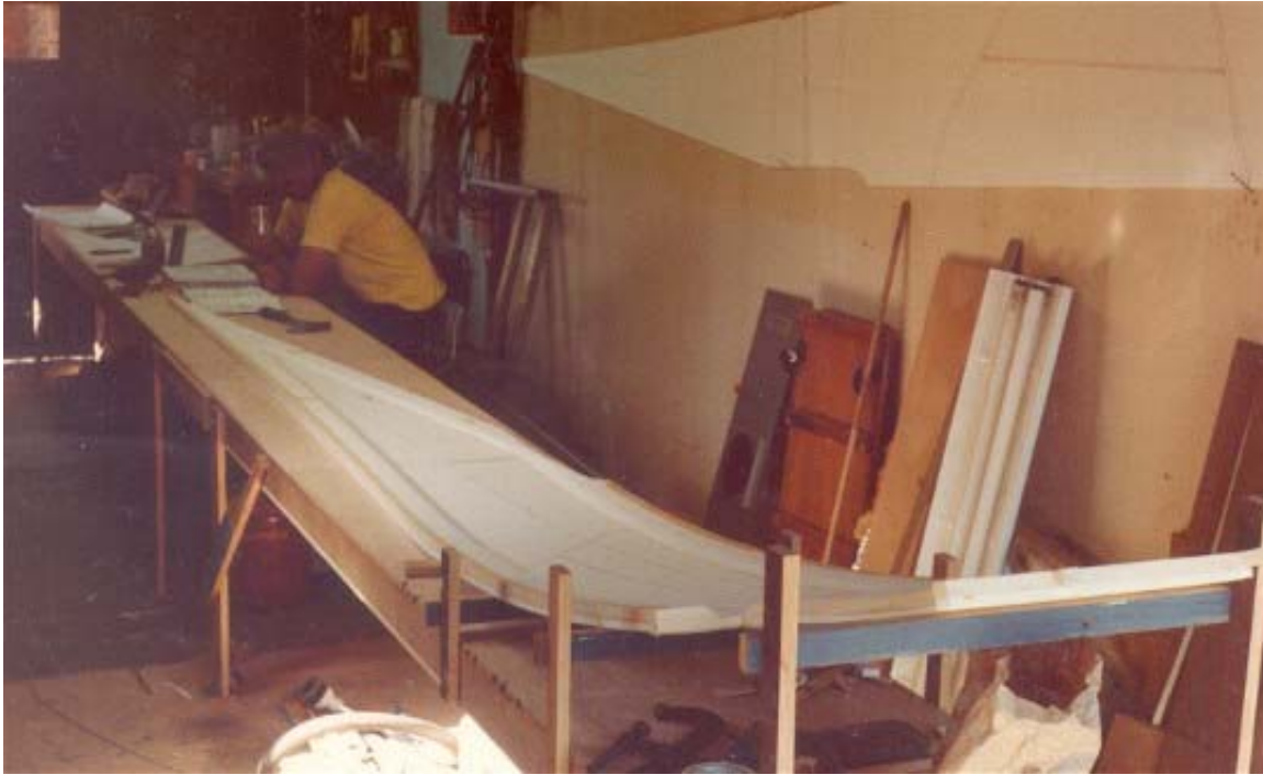
LEFT SIDE READY TO GLASS, RIGHT SIDE ON WALL
